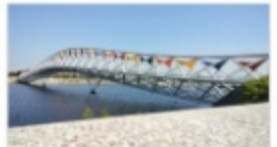
ATAL BRIDGE - AHMEDABAD
