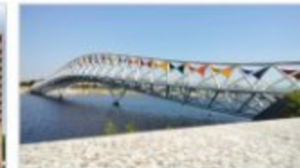
ATAL BRIDGE - AHMEDABAD
