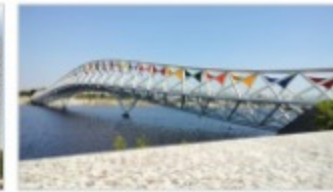
ATAL BRIDGE- AHMEDABAD
